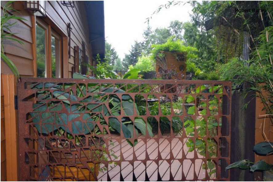
A gate leading from the back deck to one of the side decks uses what was left of a sheet of metal after machine parts were cut out of it by laser.
